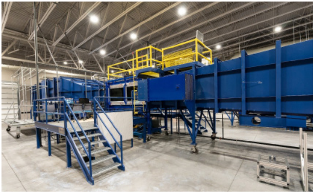
Figure 1: A view of the new ERAU wind tunnel and the test section, which sits in a dedicated 16,000 square-foot building.
